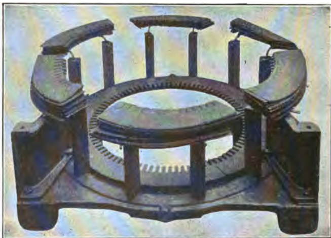
FIG. 98.—Laminations partly assembled, making up the armature core of a skeleton frame alternator.
